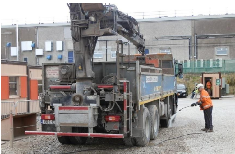
Figure 5.5 – Example of wheel washing of truck as it leaves site
